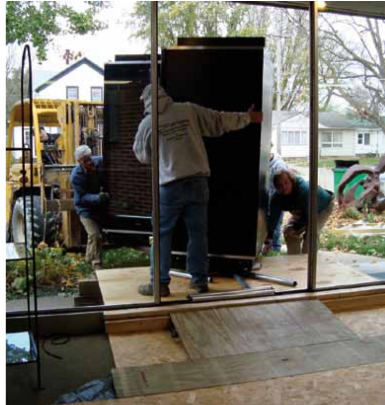
The new inside wrap cooler had to be brought in through the front windows. The center pane was removed with literally an inch to spare on each side. The crew wiggled it through the narrow opening.
