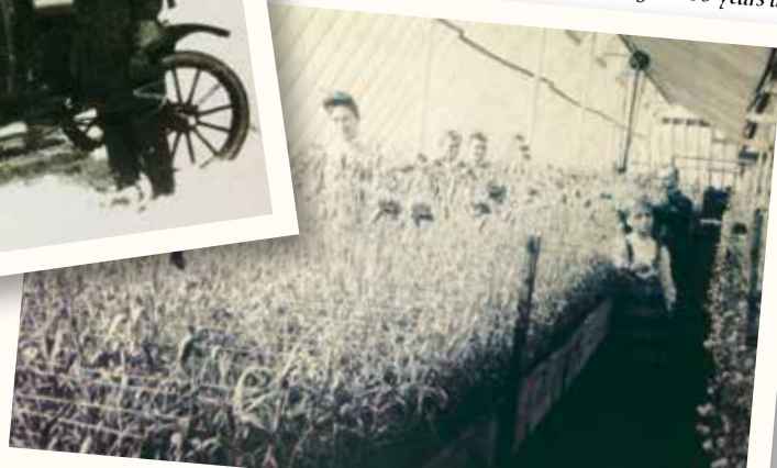
The old greenhouse where the business began 135 years ago.
